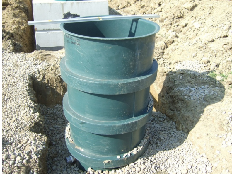
Figure 5. Dosing siphon - external view
