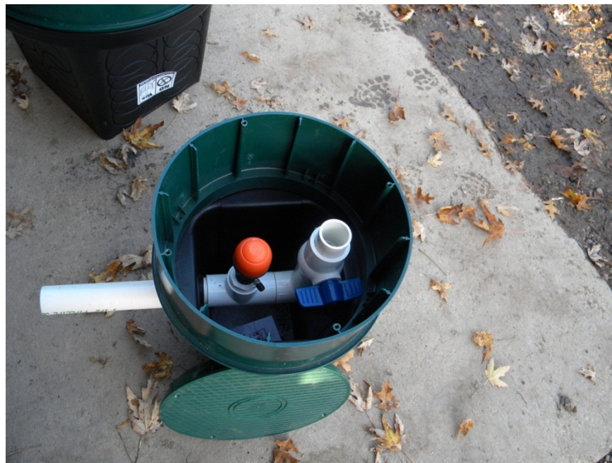
Figure 8. Turn-up and \frac{3}{4} inch air gap/ bleeder at the end of each lateral for routine maintenance
